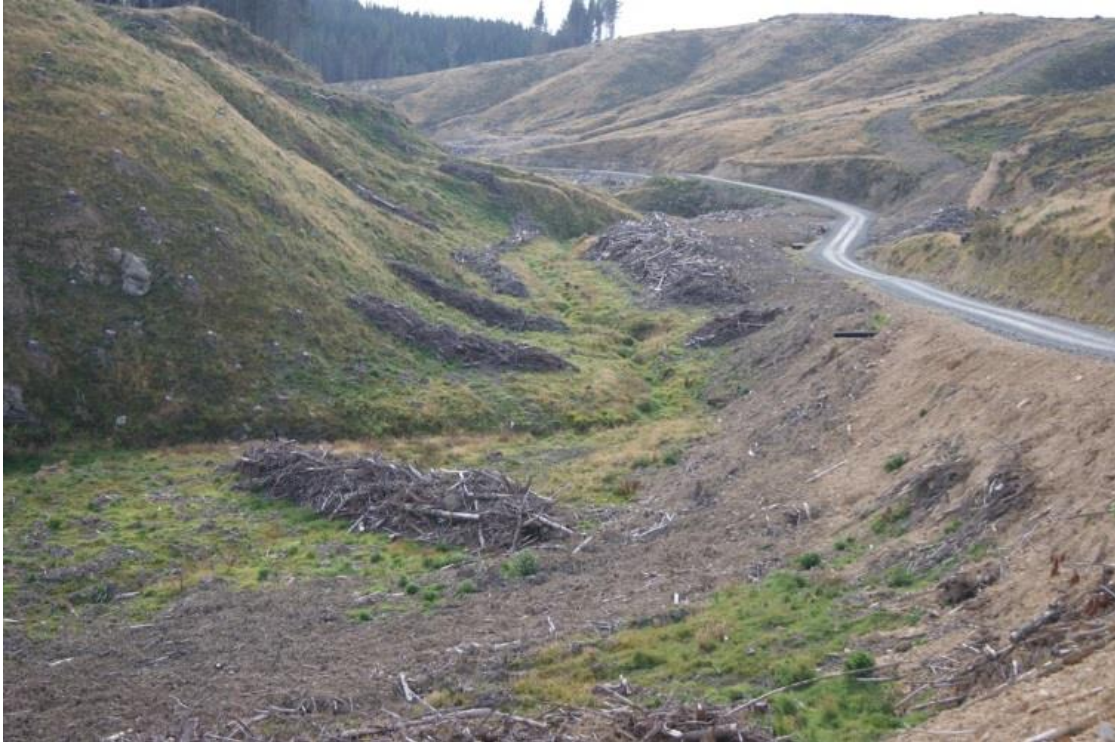
Figure Three - Overview of creek position in relationship to the road, wind rowing and forest harvesting. Note the available width of the area.
